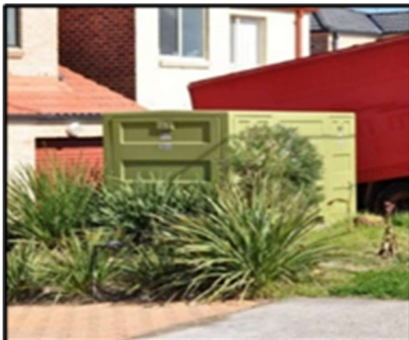
Padmount substation
