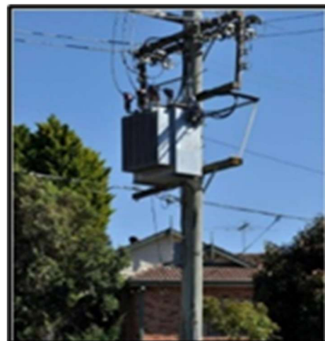
Pole mounted substation
