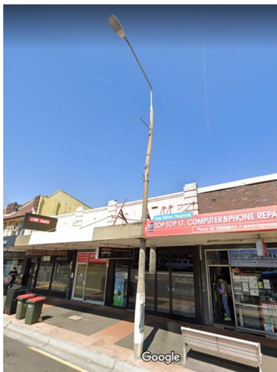
The street awning is inappropriately constructed around the streetlight column. Source: Google Maps Street View.
